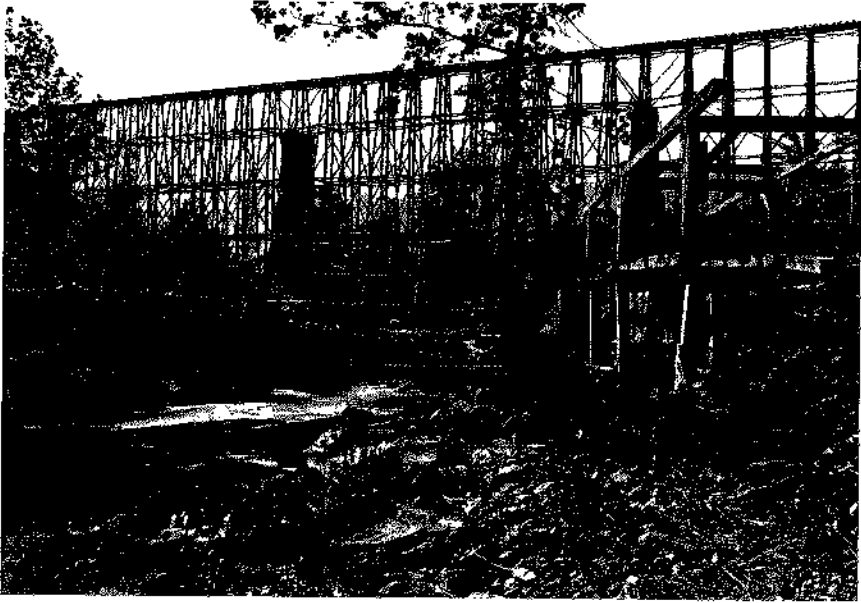
FIGURE 12. "Trestle Bridge at Whiteside" (Barnard, Plate 4).
